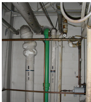
The soft water main runs from the three water softeners in the boiler room to the tunnel washers at the back of the facility. It is a run of approximately 400 feet.
